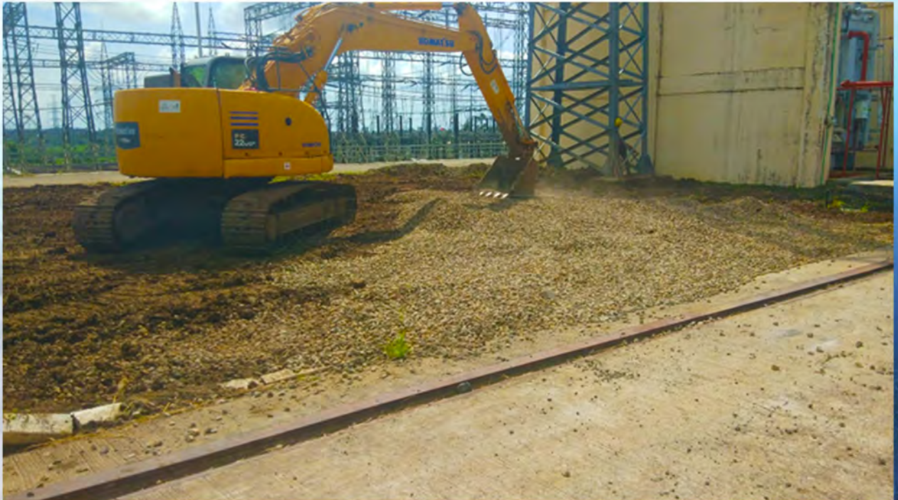
Leveling and Gravel Bedding of TN-C2
