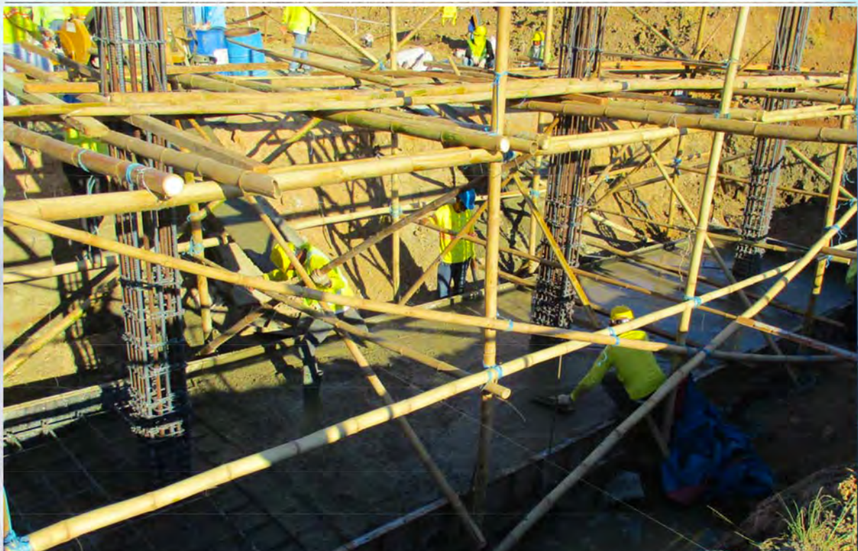
Concrete Pouring on PTR's Firewall Combine Footing
