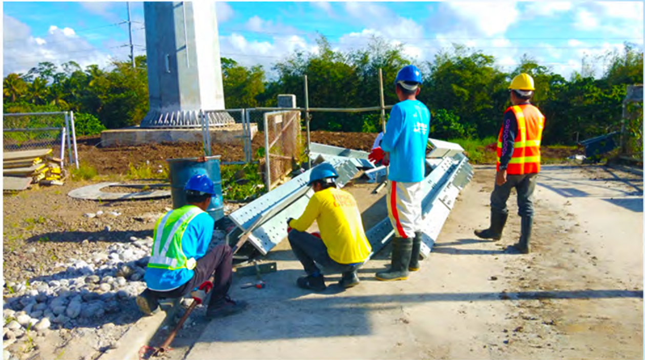
Preparation for Stub Setting
