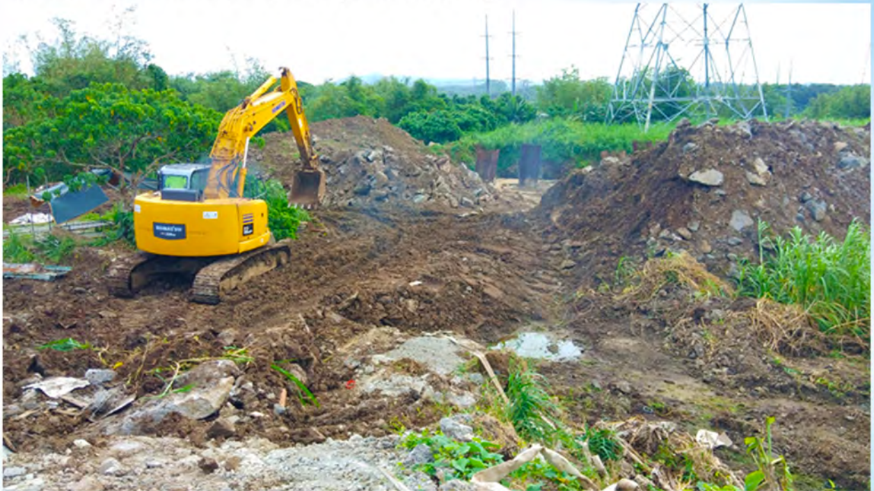
Preparation of Access Road for TN-A1
