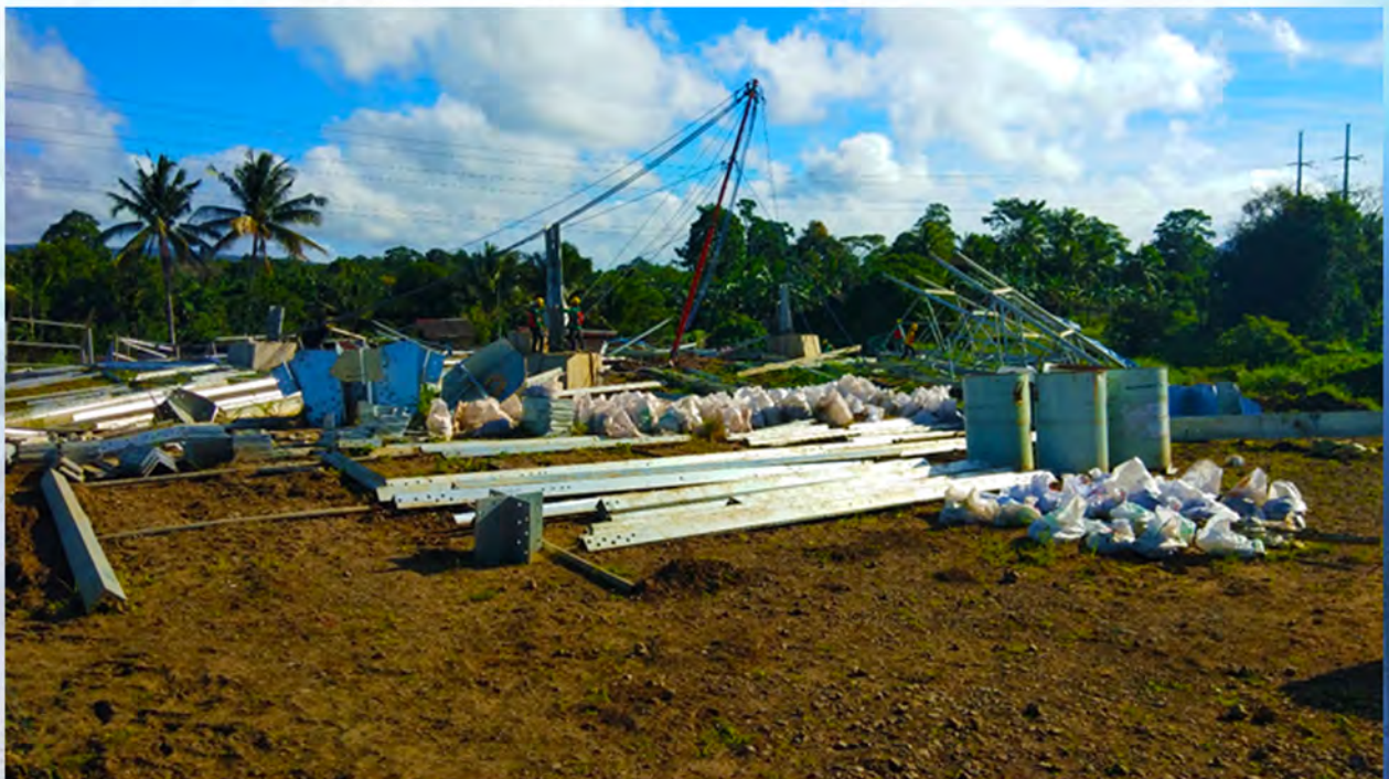
Segregation of Tower Parts and Repairing of Steel Pole Ladder
