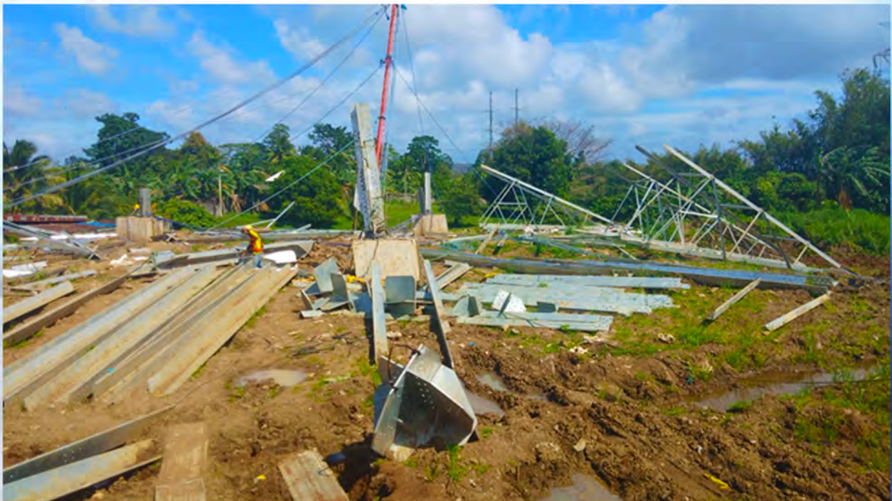
(TN-B1)- Segregation of Tower Parts
