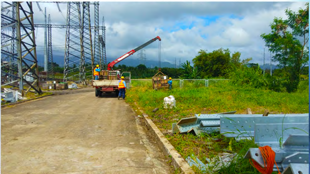
Hauling of Insulators
